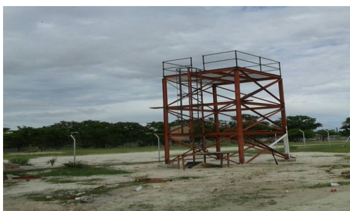
Fig.2 Construction of Oshakati Constituency Office Water Tank, Oshana Region
