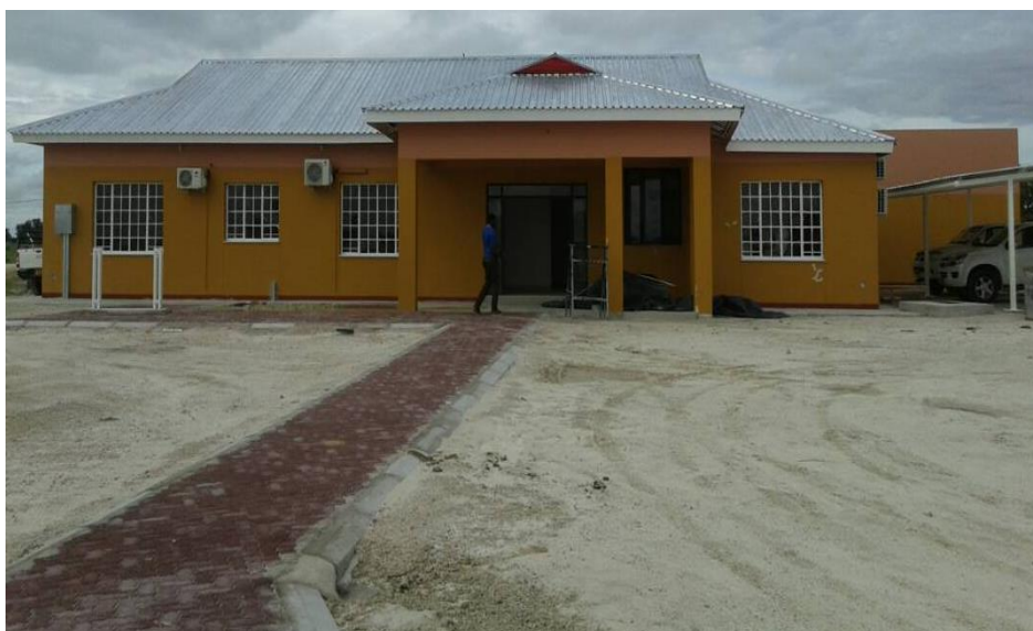
Fig.1 Construction of Oshakati Constituency Office, Oshana Region
