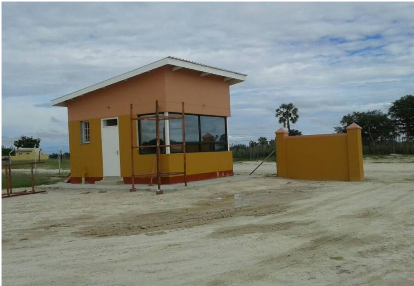
Fig.3 Construction of Oshakati Constituency Office Guard House, Oshana Region
