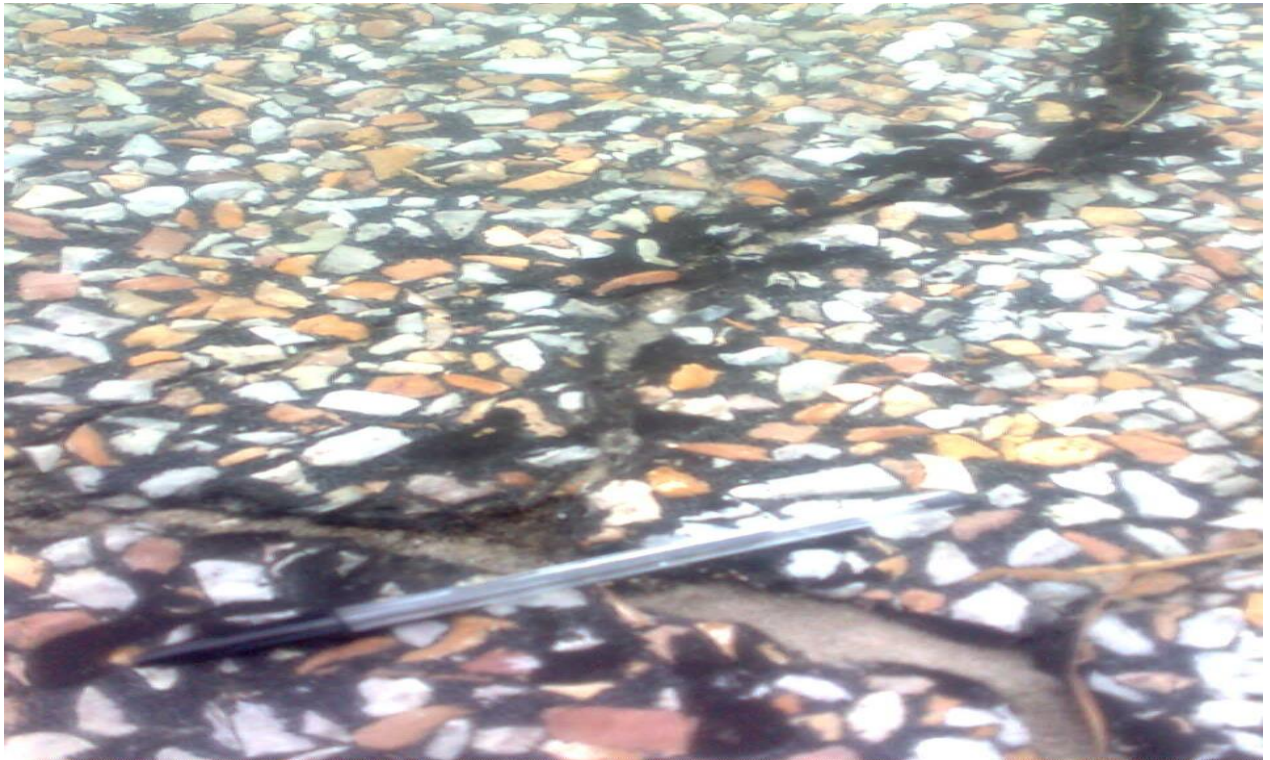
Cracks on Katima Mulilo Aerodrome Runway
