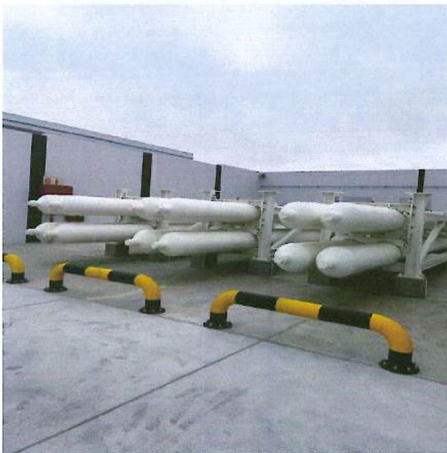
<<< Storage Cylinders for hydrogen
