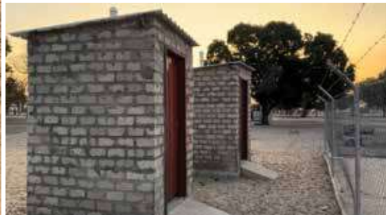
Ablution facility at an open market in Kavango West Region
