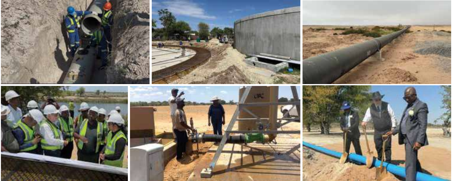
Construction of Water Supply Security Infrastructure Projects
